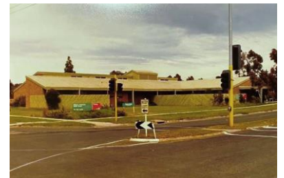
Sunbury Community Health Centre in its original location (now Hungry Jacks). PTO for further info.
