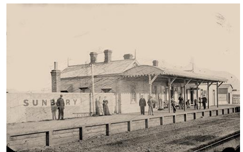
Sunbury Station (1 of 4) c. 1860s (oldest known photo)
